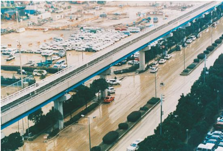
Liquefactions caused by the Southern Hyogo Prefecture Earthquake (photos: Kobe City)
