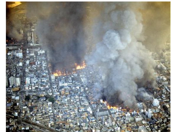
Damage in Kobe City (photos: Kobe City)
