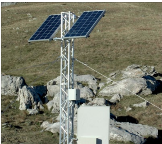
Fig. B - Automated Inclinator System (AIS) installed in the El Portalet active landslide.
