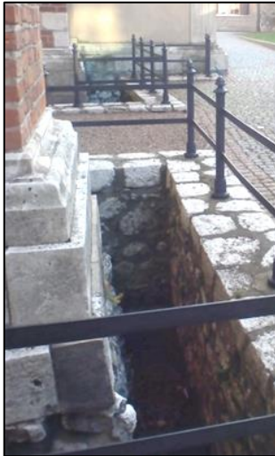
Photo 2. Narrow depression around the walls of an old church representing the former ground level (Phot. R. Zarychta).
